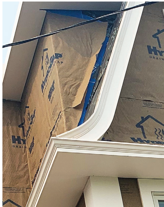
After cooling, the trim retains its curved form (left). For this project, crown molding was used to provide the flared edge common on many homes designed in Dutch Colonial and Tudor Revival styles (right).
