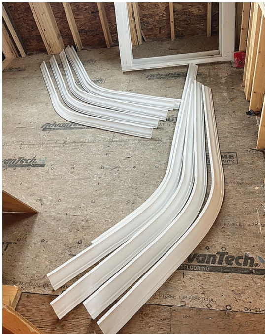
After cooling, the trim retains its curved form (left). For this project, crown molding was used to provide the flared edge common on many homes designed in Dutch Colonial and Tudor Revival styles (right).
