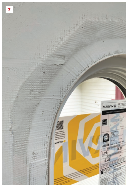
The first coat was done with Durabond-90 joint compound. At the gap between the jamb and the drywall, the author pushed Durabond through the mesh about 1/2 inch to key it in (7). Three coats of USG Plus 3 joint compound were used to blend and float the edges out. The completed trimless return (8).
