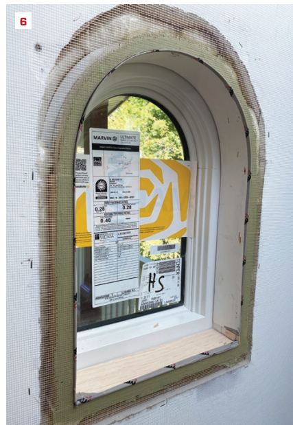
A temporary screed board (its edges wrapped with plastic tape for easier release) was run 1/4 inch proud of the jamb extensions (5). To avoid overlapping seams and the potential for cracking, a single piece of mesh was installed, cut to the opening, and set in liquid-applied Hydro Ban waterproofing (6).
