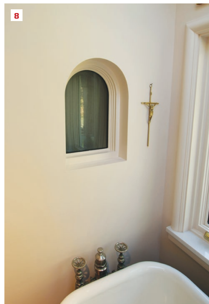
The first coat was done with Durabond-90 joint compound. At the gap between the jamb and the drywall, the author pushed Durabond through the mesh about 1/2 inch to key it in (7). Three coats of USG Plus 3 joint compound were used to blend and float the edges out. The completed trimless return (8).
