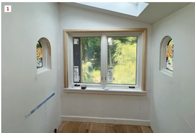
The homeowners requested a plaster-like interior finish for a pair of small, arch-top windows in their bath remodel (1).
