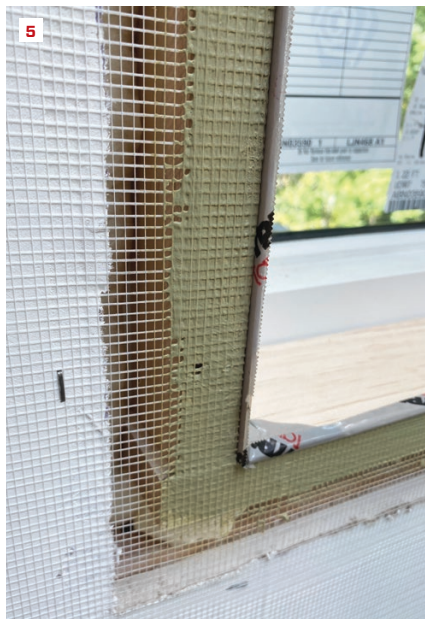
A temporary screed board (its edges wrapped with plastic tape for easier release) was run 1/4 inch proud of the jamb extensions (5). To avoid overlapping seams and the potential for cracking, a single piece of mesh was installed, cut to the opening, and set in liquid-applied Hydro Ban waterproofing (6).
