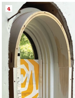
The homeowners requested a plaster-like interior finish for a pair of small, arch-top windows in their bath remodel (1).
