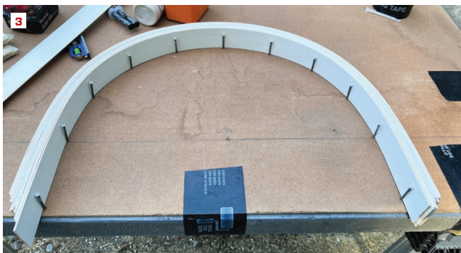
The arched portions of the jamb extensions were made from thin strips of pine bent and glued up in a site-built form (2, 3). The finished assemblies were glued and screwed flush to the window frames (4).
